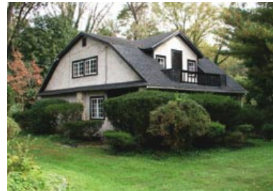
“The house of the democrat,” a two-storey stucco bungalow with dark, damp cramped interiors designed by Will Price and built in Rose Valley, PA
